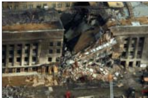
West wing: The damage to the Pentagon.
